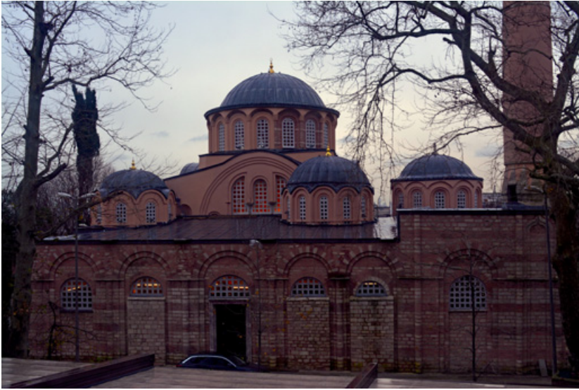
Figure 10 The Chora Church, view from the West. Photo: Dimitra Sikalidou
