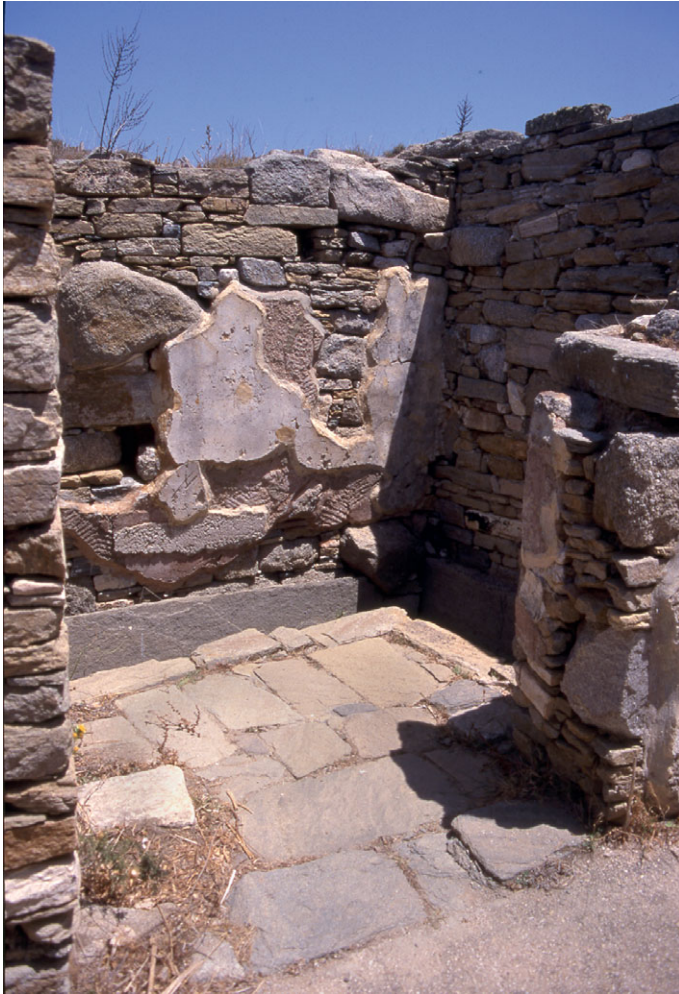
Figure 1.2 Toilet showing the paved floor with the water channel behind. Delos, Hermes House.
