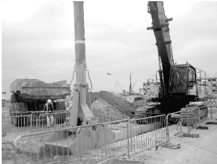
Figure 3. Possible disturbance to the under-slurry filter cake by the digging tool.
