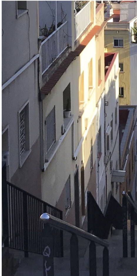
Figure 12. Dipòsit 10 in 2023 (authors).
