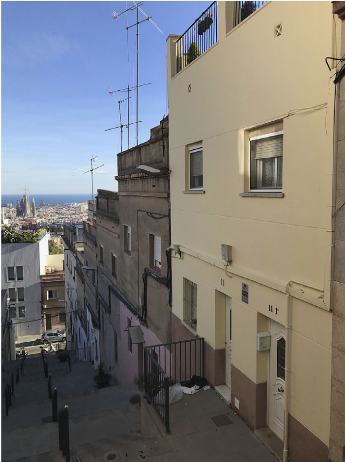
Figure 17. View of the building in 2023, more or less as in the 1955 plan (authors).
