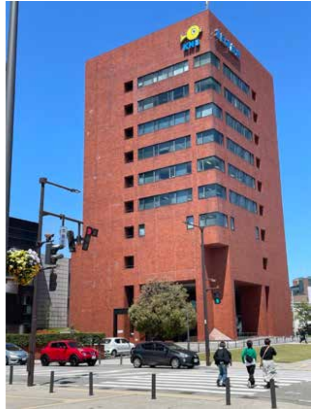
Fig. 3 KNB headquarters in Toyama City (photo by the author).
