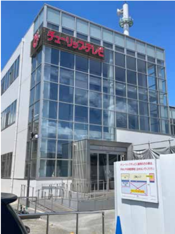
Fig. 2 Tulip TV headquarters in Toyama City (photo by the author).
