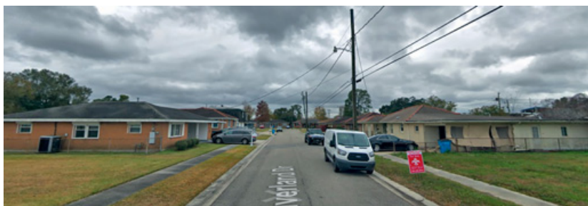
Figure 12 Typical Chalmette street.
