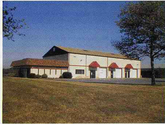
IXRF's Trenton New Jersey facility
