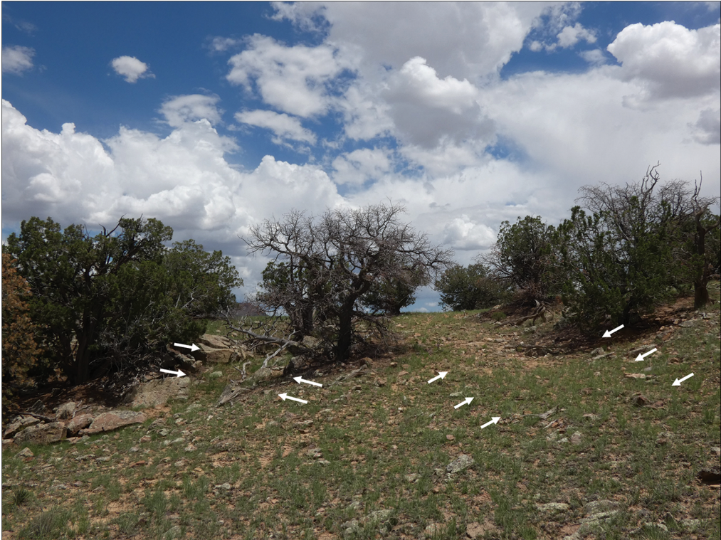
Figure 6. Fork on the Gasco South Parallel Road. The left fork passes through a natural gap in a sandstone outcrop, and the right fork is a constructed cut-and-fill segment (figure by Robert S. Weiner).
