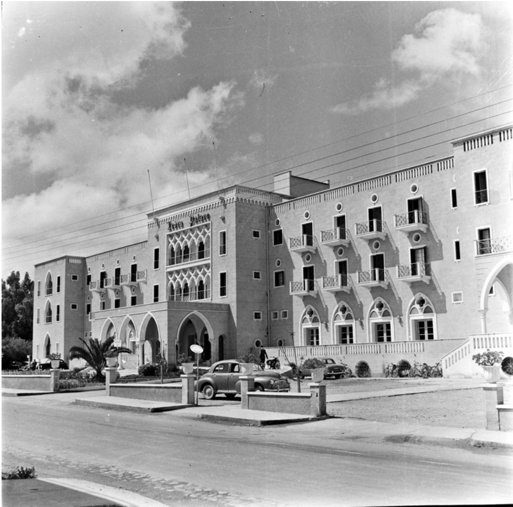
Fig. 2. The Ledra Palace Hotel in the 1950s (Photograph by Felix Yiaxis, Press and Information Office Photographic Archive, Nicosia, Cyprus)
