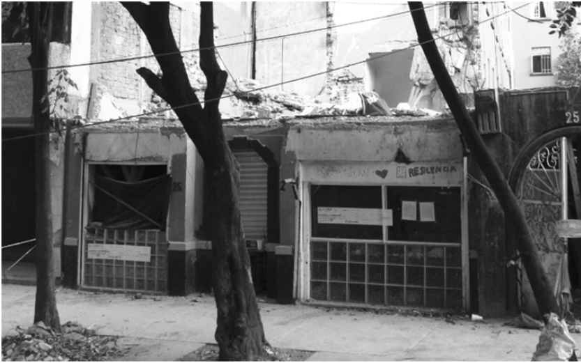
Figure 1.2 Remains of a building in Mexico City after the September 2017 earthquake. The painting on the wall reads “Juan ♥ resiliencia.” (Note from the author: the correct spelling for this term in Spanish is resiliencia . This mistake was probably due to the fact that resiliencia is a new term in Spanish.)
