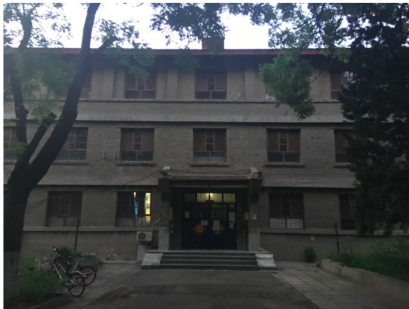
Old dorm slated for demolition
