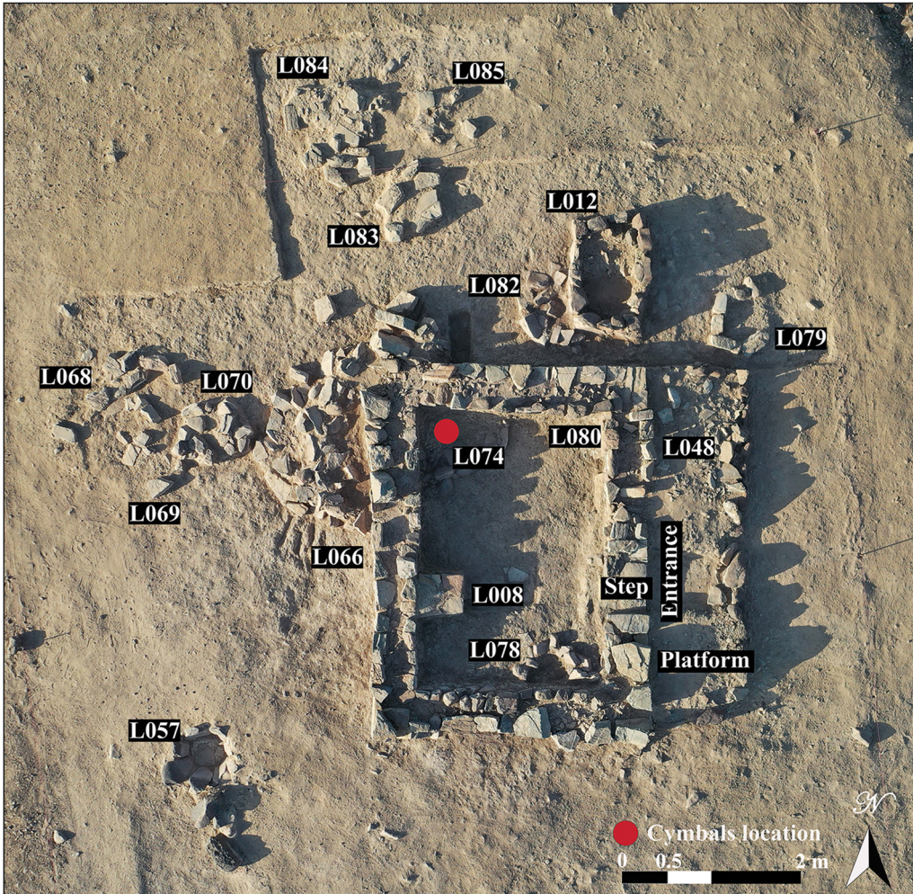
Figure 3. Drone image of building S1 taken at the end of the 2021 field season (photograph by S. Al-Mamari).
