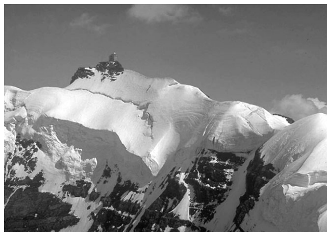
Fig. 1. The ice crest on the Sphinxgrat, Jungfrauoch, from the north, with the astronomical/meteorological observatory on the (permafrost-) rock summit, before construction of the new restaurant. (Photograph taken from helicopter by W. Haeberli, July 1986.)
