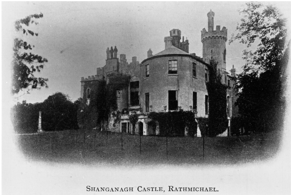
Fig 10. Castle Shanganagh with Cockburn's monument to the 1832 Reform Bill visible on the far left of the photograph. Photograph : © Irish Architectural Archives.
