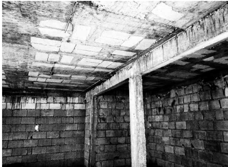
2 Chalky limestone aggregates used in construction in Port-au-Prince, Haiti, in 2012 seen two years after the devastating earthquake of 2010.
