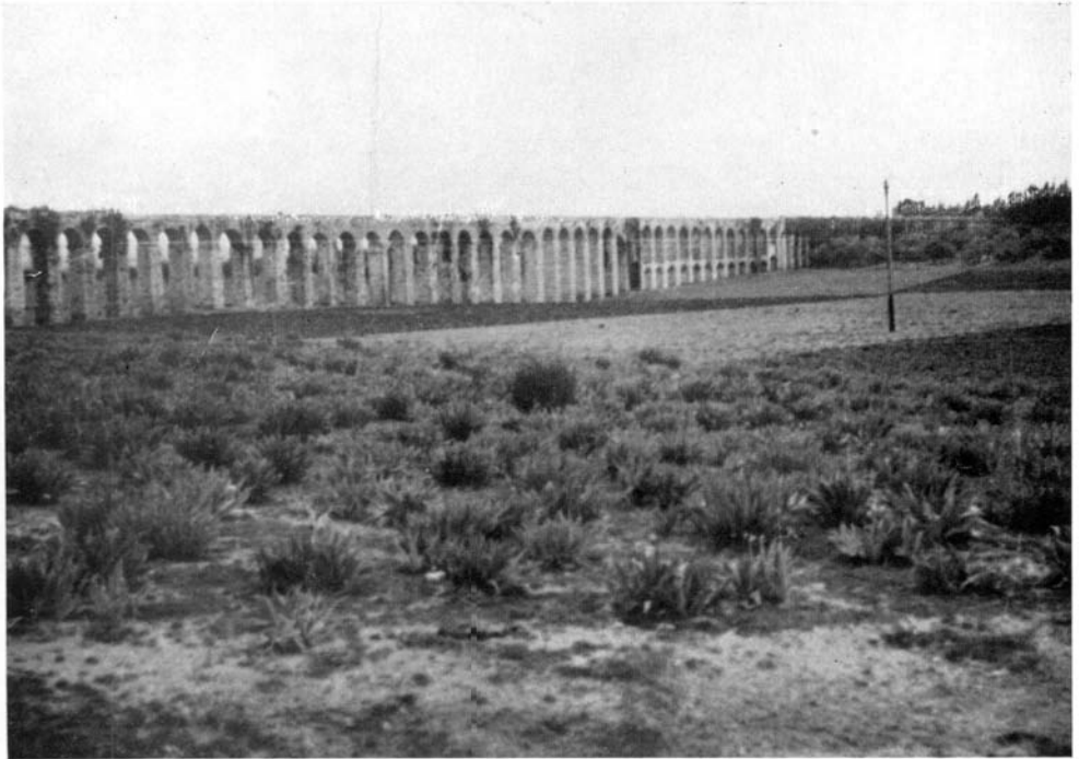
The Al Kabiri aqueduct.
