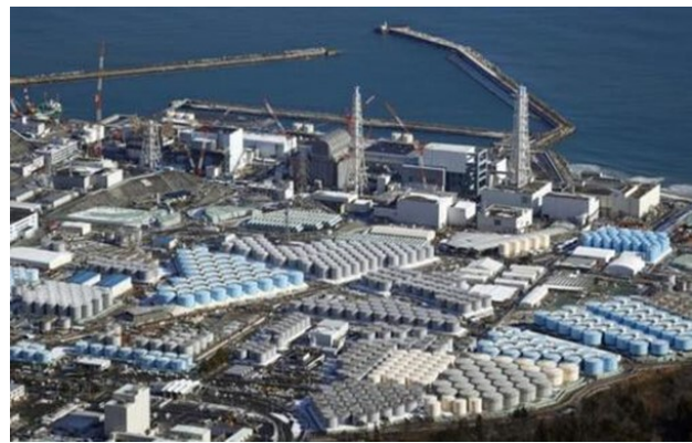
Water Storage Tanks at Fukushima Daiichi Credit: TEPCO
