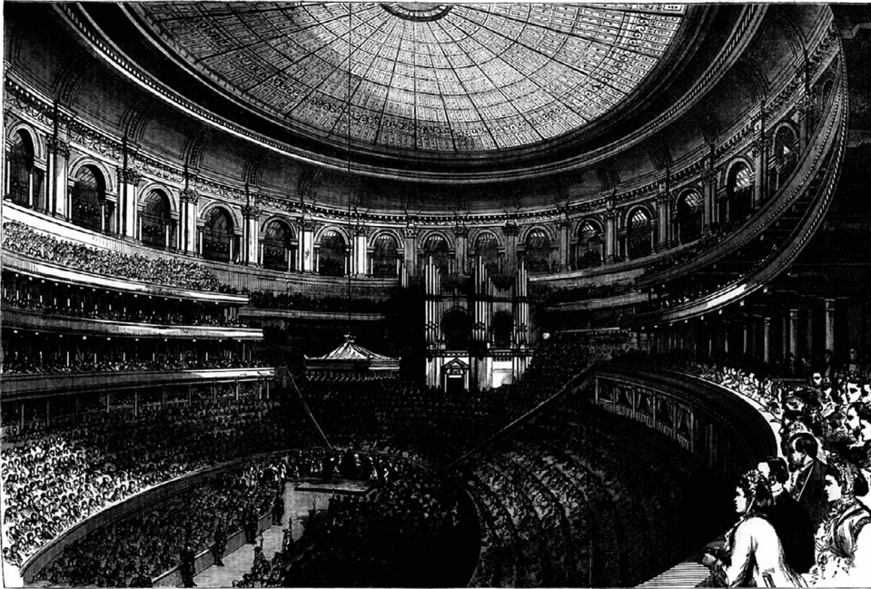
Figure 3. Opening of the Royal Albert Hall on 29 March 1871, Illustrated Times , 8 April 1871. The image shows the glazed roof, which was in reality shielded by the calico velarium designed to prevent glare and dampen resonance. Newspaper image © The British Library Board. All rights reserved. With thanks to The British Newspaper Archive ( www.britishnewspaperarchive.co.uk ).
