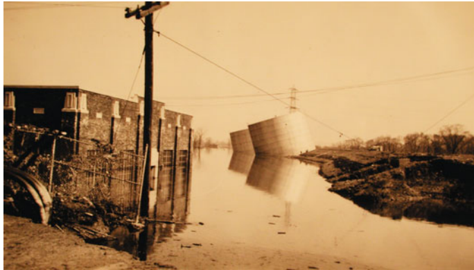
FIG. 2. Photograph of oil tanks tilted by floodwaters near a commercial building in Hartford, taken by Thomas F. Oakes in March 1936. Connecticut Museum of Culture and History, accession no. 2001.21.12.
