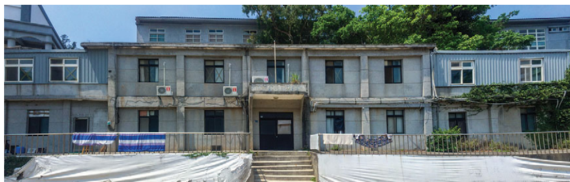
Fig. 4.1 The main building of the Supply Cooperative (Photo by the author)
