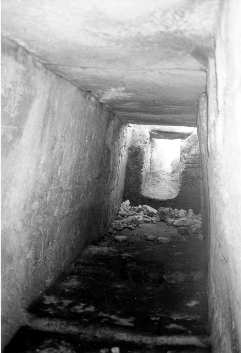
Figure 4. The interior of the dolmenic hypogeum of Le Castellet , Fontvieille. The floor, side-walls, entrance and ramp in the photograph have been excavated out of the bedrock, but the roof is formed of slabs. Note the extraordinary care with which the various components have been shaped, and the near-perfect fit between adjacent roof slabs. (Photograph by M. Hoskin).
