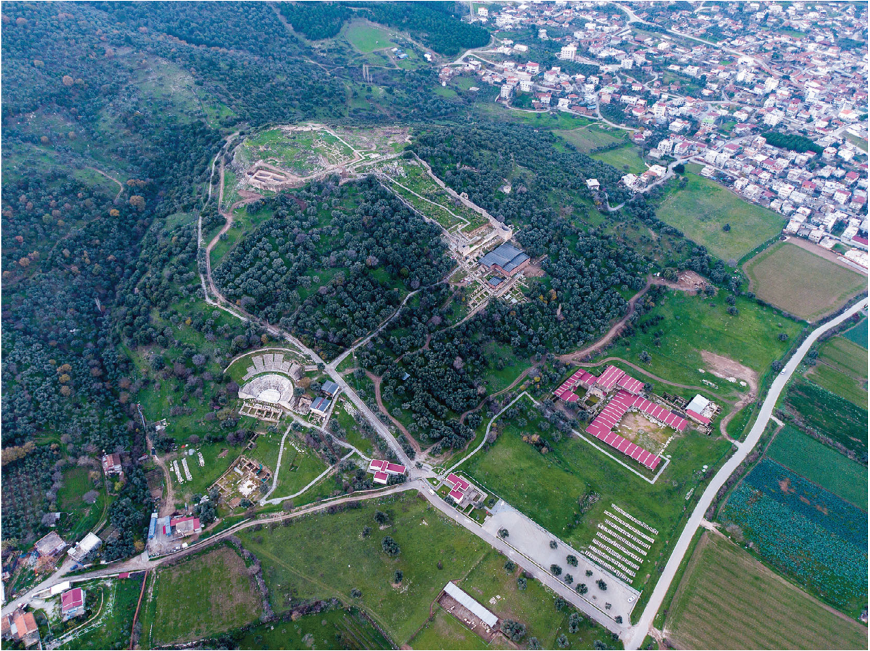
Figure 1. Aerial view of Metropolis (© Metropolis Excavation).
