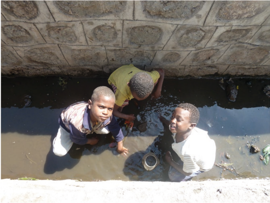
Figure 2. Young children playing in culvert, Hawassa
