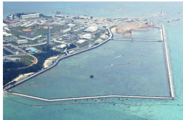
Henoko base construction
