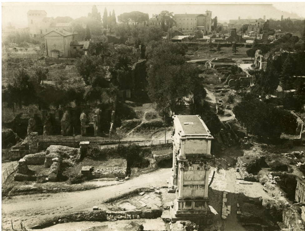
Fig. 33. In the foreground: the Arch of Titus. In the background: Villa Smith and the expansion commissioned by the Sisters of Visitation. Detail from unknown photographer active in Rome, Veduta aerea dell'arco di Tito e del Palatino , 1924, silver bromide gelatin print. Rome, MR, Archivio Fotografico, AF — 3790. Courtesy of the Sovrintendenza Capitolina — Museo di Roma.
