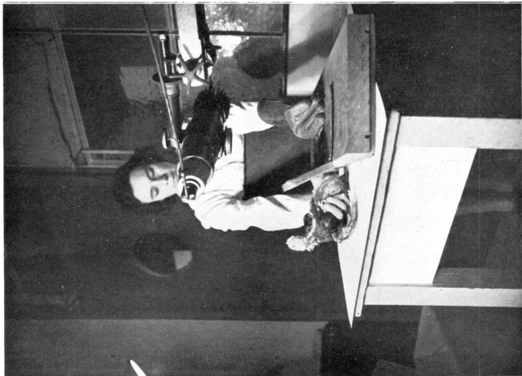
Fig. 4. Apparatus for radiographing chicks, showing lead protection.
