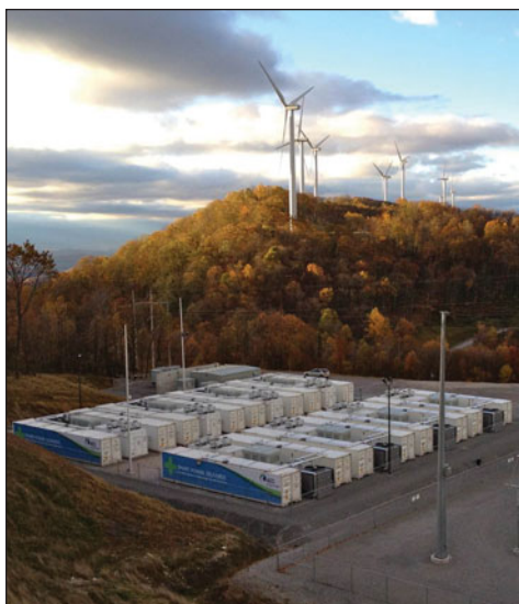
A 32 MW fleet of batteries smooths the output from the AES Corporation's wind farm in Laurel Mountain, W.Va. Image courtesy of AES.
