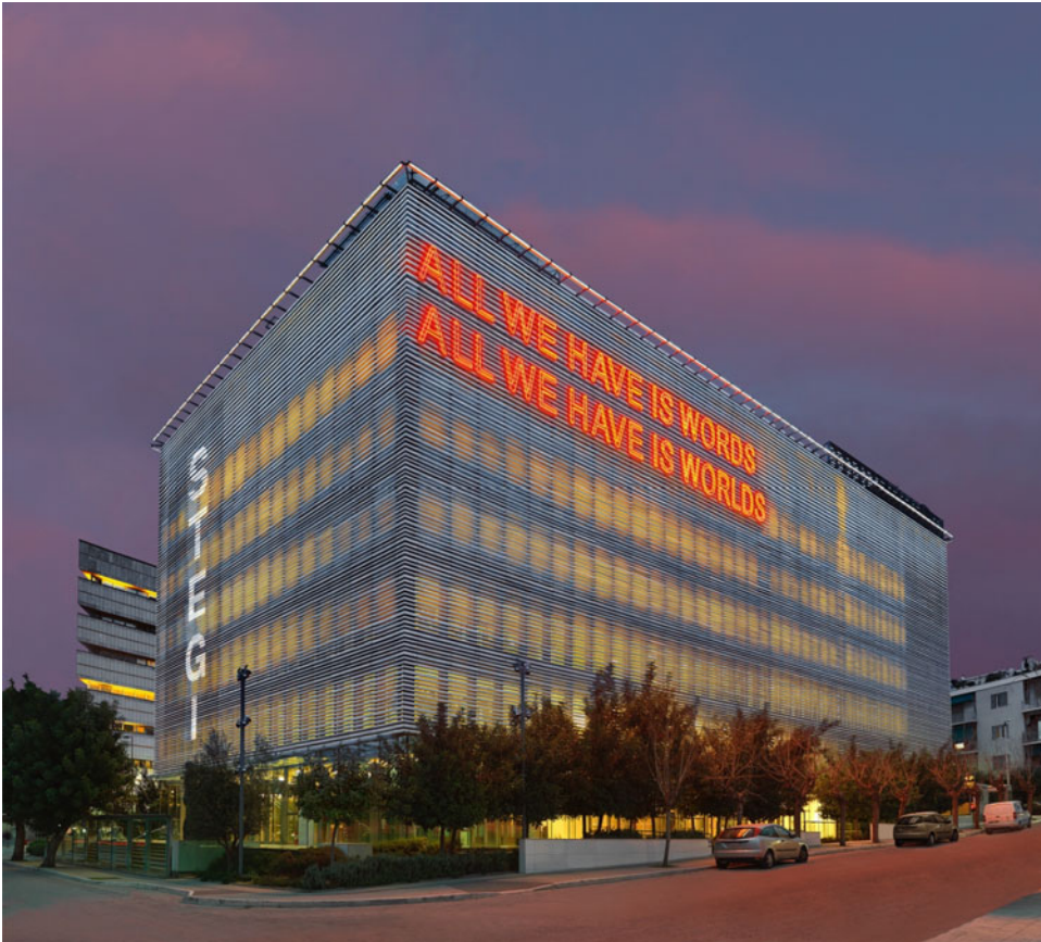
Fig. 2 Onassis Stegi Building | Stelios Tzetzias for Onassis Stegi
