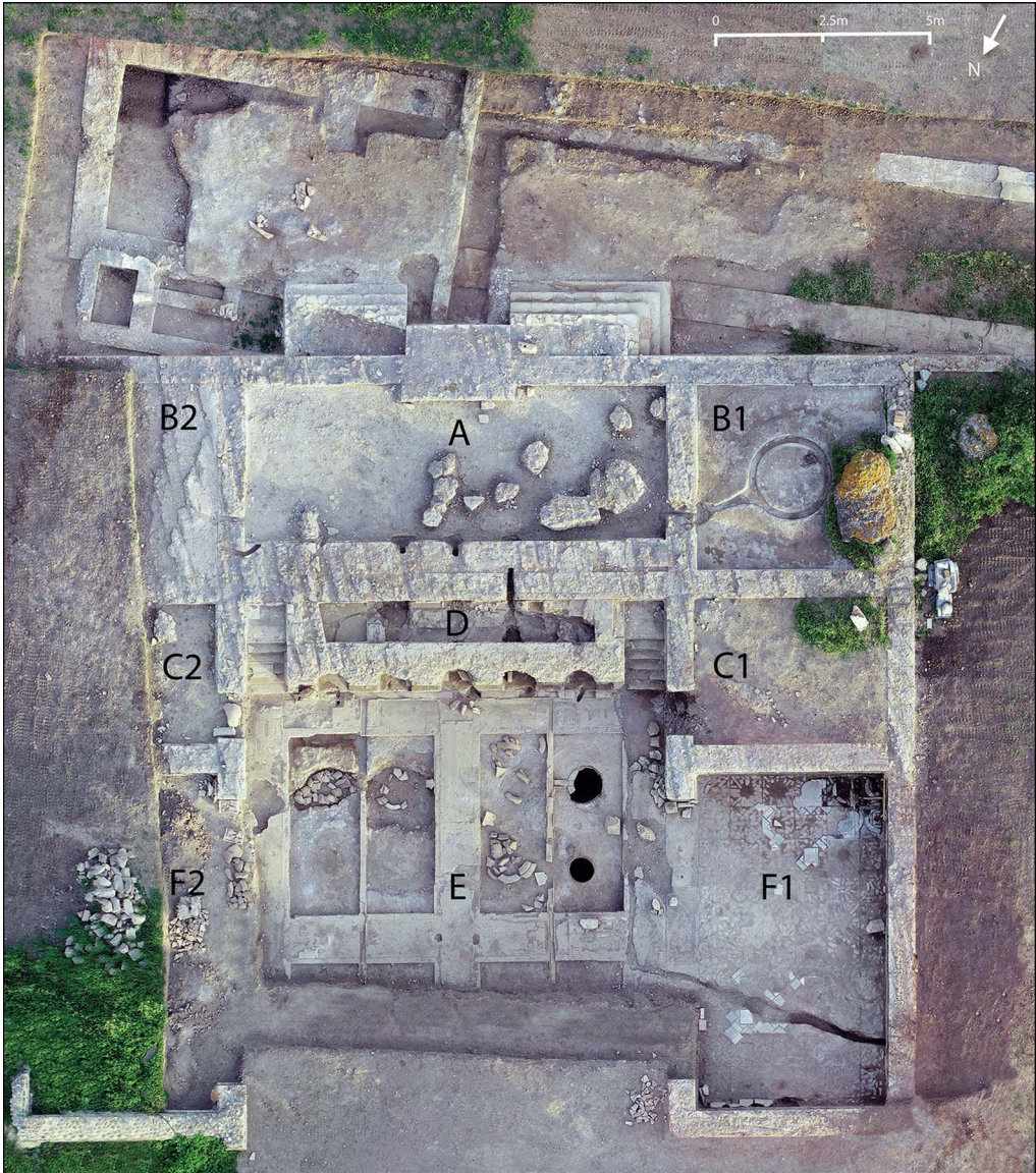
Figure 2. Aerial orthophotograph of the Villa of the Quintilii winery building, indicating the treading area (A), press beds (B1 and B2), proposed press mechanism rooms (C1 and C2), collection vat (D), cella vinaria (E), and dining rooms (F1 and F2) (image by M.C.M s.r.l, modified from Frontoni et al. 2020: fig. 3).
