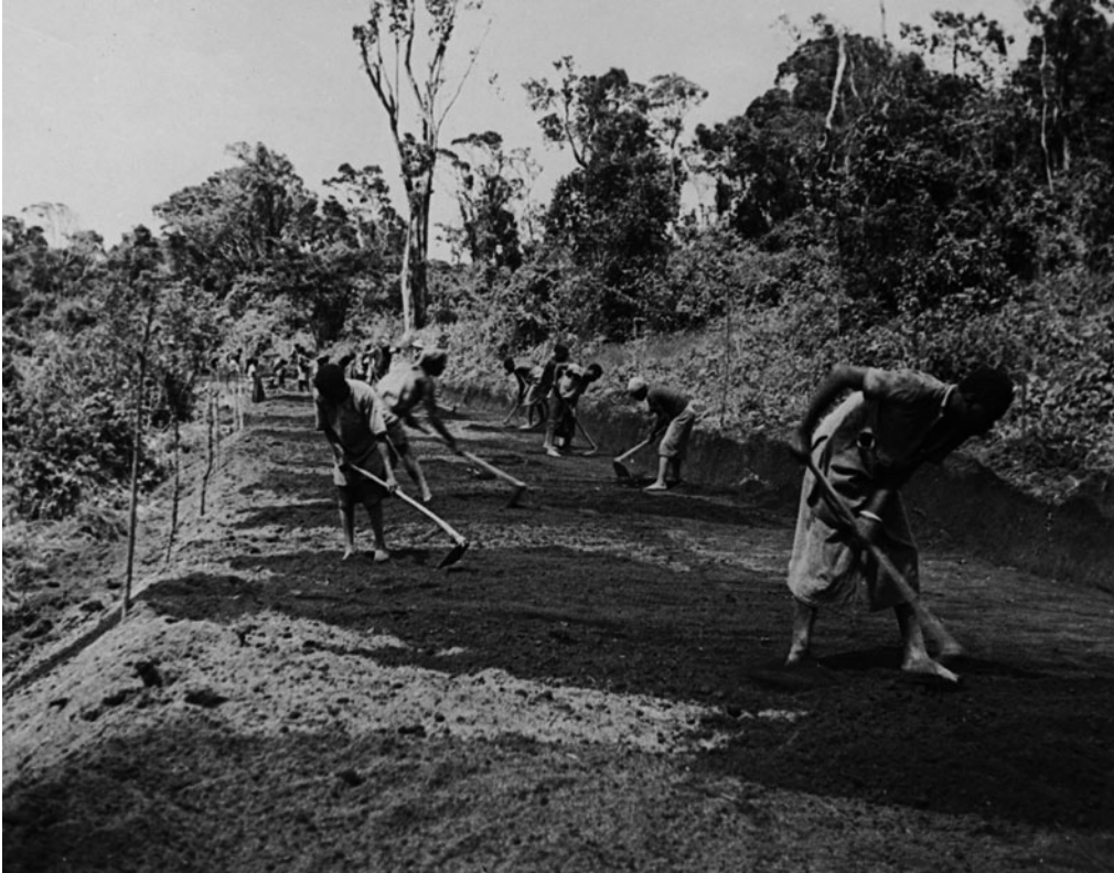
Fig. 2. Ocker, 'Road construction in Mufindi', n.d.
