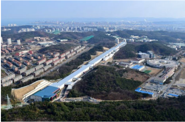
Figure 1. Construction site of PAL-XFEL.
