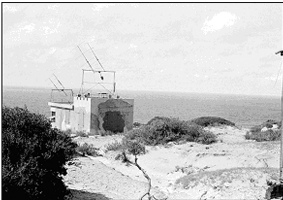
Figure 4 The War-era blockhouse, with 100 (left) and 60 MHz (right) twin Yagi antennas mounted on the roof. The 200 MHz 4-Yagi antenna which was located on the seaward right-hand corner of the blockhouse is not readily visible in this photograph (ATNF Historic Photographic Archive: 1031–3).
