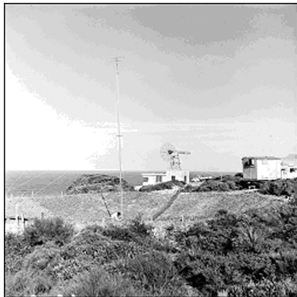
Figure 13 View of the prototype hole-in-the-ground antenna, looking towards the blockhouse (ATNF Historic Photographic Archive: 2763–2).
