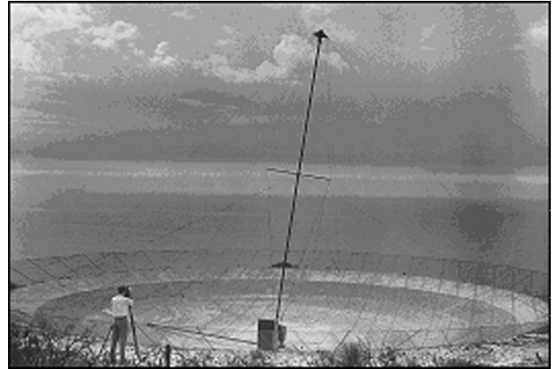
Figure 14 The 24.4-m hole-in-the-ground antenna, with Gordon Stanley surveying the position of the aerial mast (ATNF Historic Photographic Archive: 3150–2).
