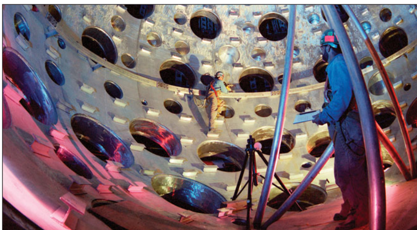
Target chamber at the National Ignition Facility, the cornerstone of the US Stockpile Stewardship Program. Credit: Lawrence Livermore National Laboratory.
