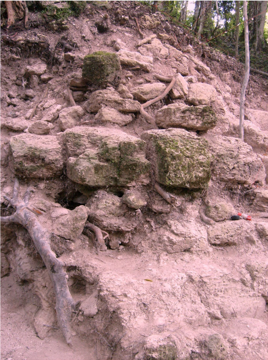
Figure 6. Destroyed mask on the east side of the fifth phase of Structure 9 (photograph by Kaitlin R. Ahern).
