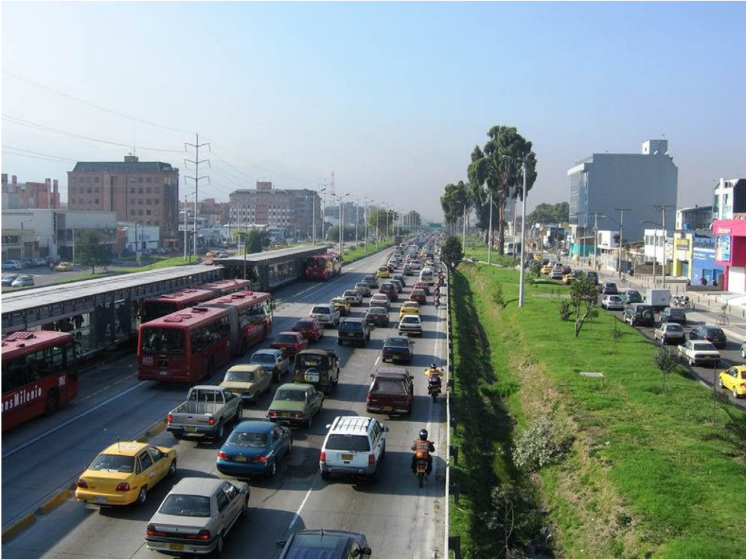
Figure 8. TransMilenio BRT – Bogotá. Source: EMBARQ (Global BRT Database, 2023).
