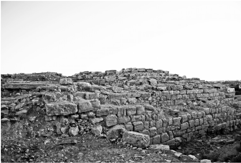
Figure 14 Southeast corner of Dhiban’s fortification system looking east. The lowest courses date to the first millennium BCE with Classical and Islamic structures built above them. This area has seen excavation and cleaning in recent years (Image: B. Porter).
