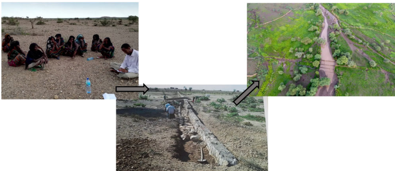
Fig. 3. Water spreading weirs constructed in the degraded landscapes of Shekay boru, Afar, Ethiopia, and the land cover changes due to the interventions (photo credit: GIZ).
