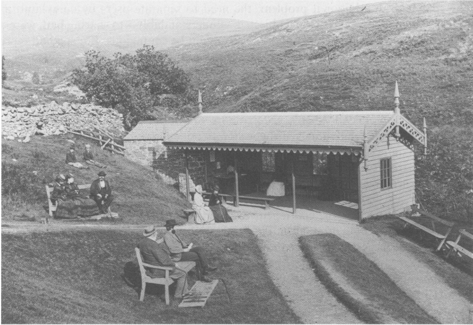
Figure 3: A view taken by the Aberdeen photographer George Washington Wilson c. 1870 of the modest well-house at Moffat with various patrons resting after their morning constitutional to take their prescribed quota of spring water. (By kind permission of Aberdeen University Library.)
