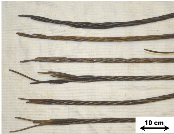
Figure 1. Macroscopic overview of broken mountain-anchors (anchor strands) made from high strength steel wires.
