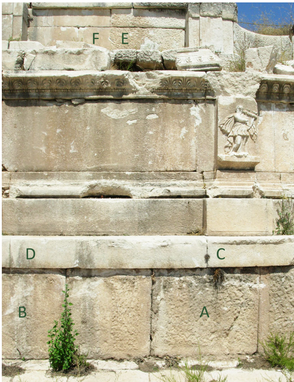
Figure 9. The Hadrianic Nymphaeum, northern wall. A) orthostats with punched dressing and pointed claw chisel-drafted margin; B) pointed claw chisel dressing; C) upper edge of the basin with punched dressing, pointed claw chisel-drafted margin, and protective flanges; D) pointed claw chisel dressing; E) rectangular niche with punched dressing; F) pointed claw chisel dressing.
