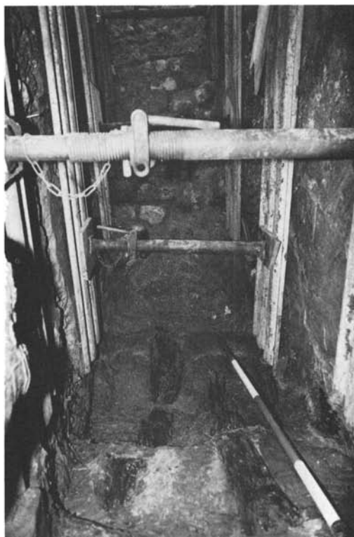
B. View of the downslope end of Trench 101 showing displaced, sub-horizontal timber piles and the displaced north wall (the scale rod is divided into 50 cm lengths). (p. 216).
