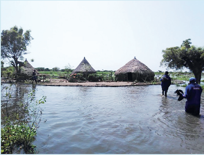
Figure Box 9.2.1 | Indigenous earth walls ( hayit ) built by Indigenous people in Akobo, Jonglei Region, South Sudan, to protect their houses and infrastructure from the worst flood in 25 years that occurred in 2019. The wall is 1–2 m high. Photo credit: Laurent-Charles Tremblay-Levesque.
