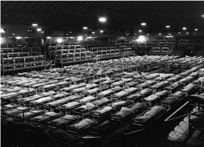
Figure 1. Men's Dormitory at Hastings Park Livestock Building, circa 1942.
