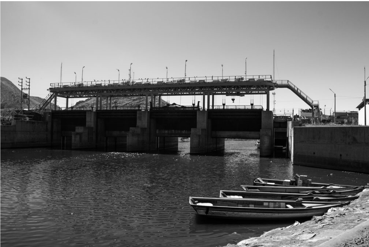
Figure 6. Dam at Desaguadero. (Photograph: S.C. Smith.)
