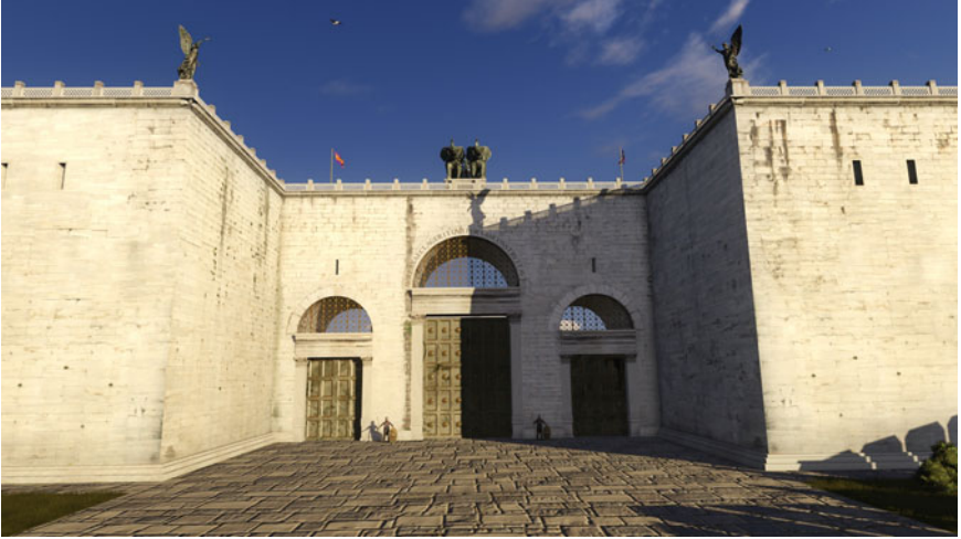
Figure 7. Reconstruction of the Golden Gate, with the figures at the bottom giving some sense of its enormous scale. The doors that obstruct the three arches were later additions (Bardill (1999) 681–3). Atop the gate is the chariot drawn by elephants (here a biga is depicted, although some sources suggest a quadriga ). Positioned on the flanking towers are Victory and the Tyche of Constantinople. © Byzantium1200.
