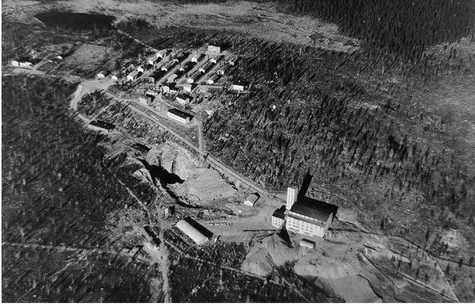
Figure 10.2 The mine and the mining settlement Laver. Credit: Boliden archives.
