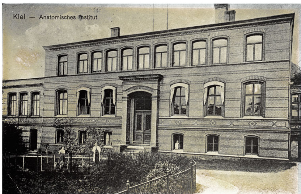
Figure 3. Photograph of a postcard of the anatomical institute in the Hegewischstraße, Kiel, as built by Gropius & Schmieden in 1878–1880, expanded in 1897 and extended further in 1901–1902. The presence of the new top floor and left wing, but not the right wing, date it to 1902–1914. The plain building, with low-pitched arches, was faced in yellow bricks with lines inlaid in red and grey: ‘Zusammenstellung der bemerkenswertheren Preußischen Staatsbauten, die im Jahre 1878 in der Ausführung begriffen gewesen sind’, Zeitschrift für Bauwesen (1879) 29, cols. 423–446, 436–437. Anatomisches Institut der Christian-Albrechts-Universität zu Kiel.
