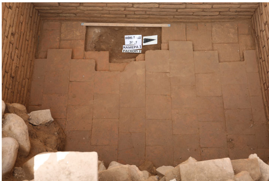
Figure 10. Floor paved with two layers of backed brick in the antechamber. Source: Photo by Kubatbek Tabaldiev and Kunbolot Akmatov.
