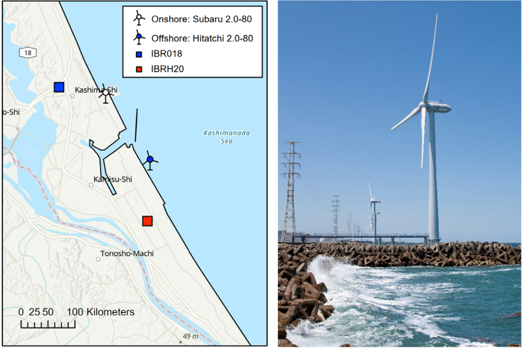
Figure 10. Photograph of the Kamisu (Hasaki) wind farm following the 2011 Tohoku earthquake.
