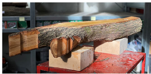
Figure 22. Structural connection: Photo of a construction element from an oak specimen, depicting the position of the contact faces of the joint, considering the central line of the tree's growth.
