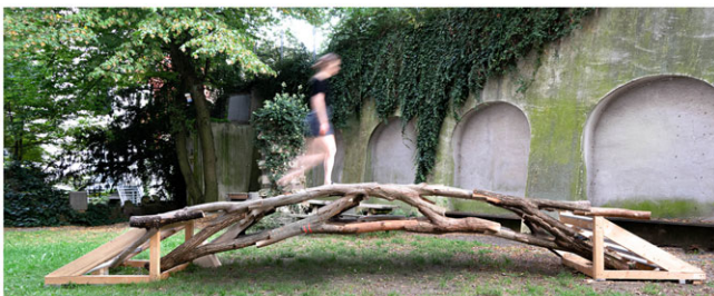
Figure 23. Final state. The construction is currently located in the inner courtyard of the Faculty of Architecture (Schinkelstr. 1, 52064, Aachen, Germany) for testing and public use.
